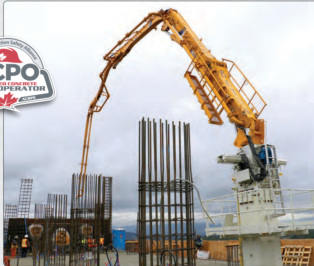
Tower placing boom in use at Surrey Central project
