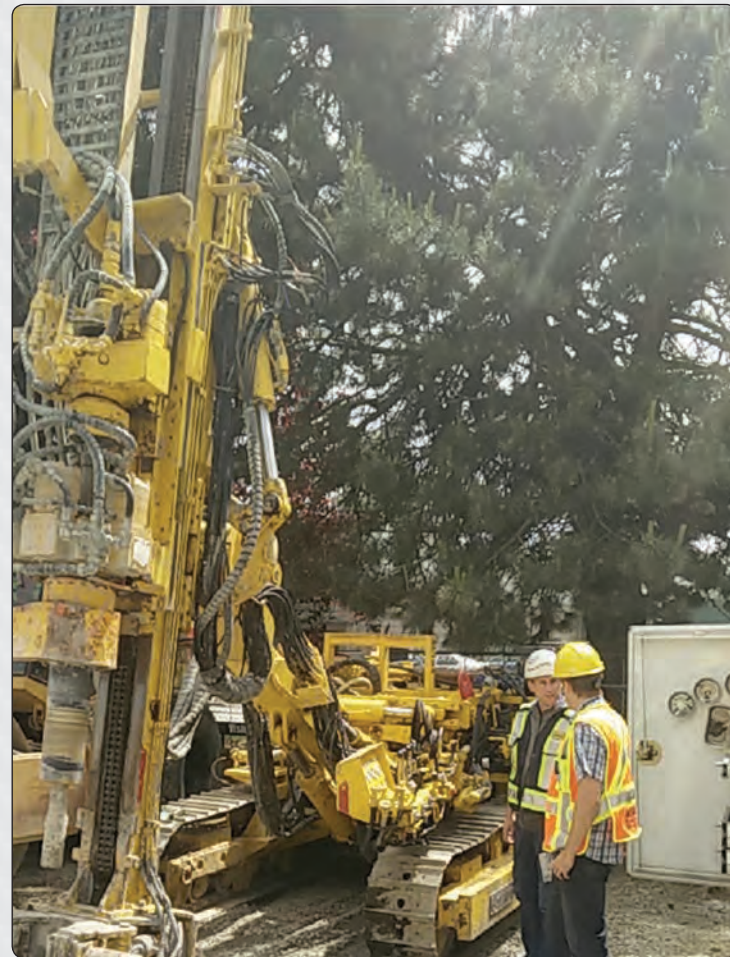
Lower Mainland RSA, Travis Robertson, consulting with local contractor, on-site
