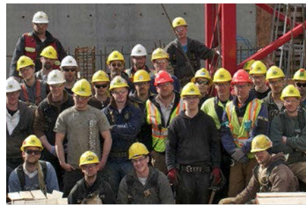
PCL's team at the BC Hydro Mount Pleasant Substation Building in Vancouver. Photo courtesy of Grant Mattice.
